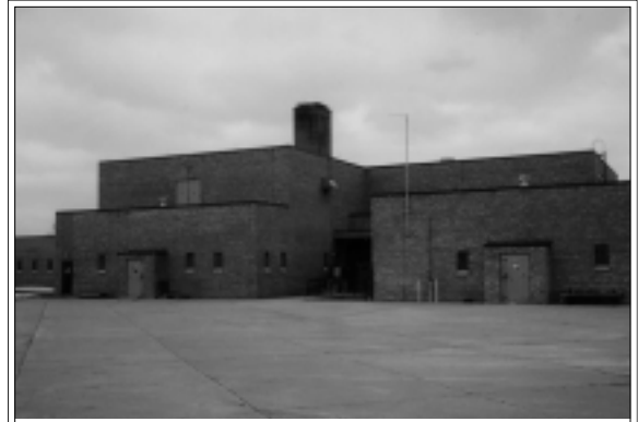
NADC Building # 3 - Animal Isolation Facility. NVSL and CVB-L lease space in this facility.
