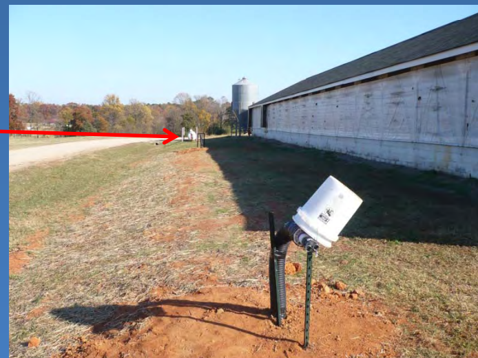
Buried Pipe (heat sink) Outlet Pipe
